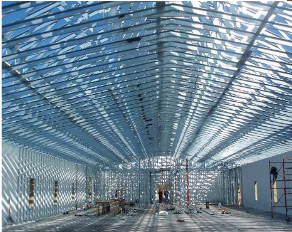
Above. Scissors roof truss system during installation.
