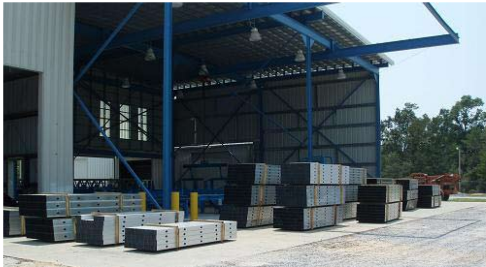
Loading zone, Freeport, FL. Lift crane for loading trusses and framing products directly to trucks.
