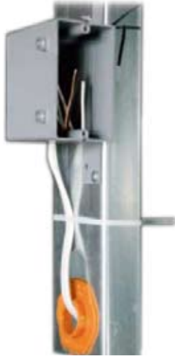
Electrical Installation on Structural Stud.
