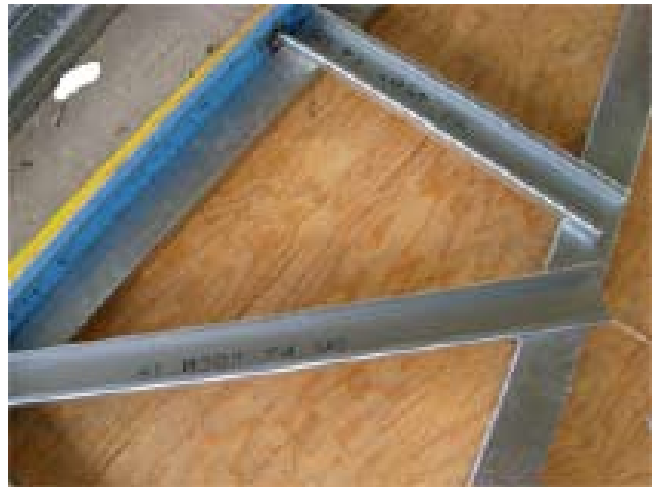
Step 2. Machine-labeled stock is placed in the jig
